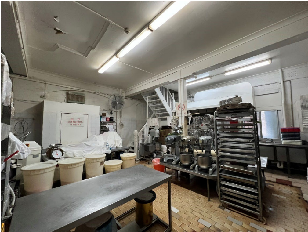
Figure 44 Industrial kitchen fit out on first floors of 98 and 100 Hay Street with its exposed beams and supporting post. The original timber staircase is in the background.
