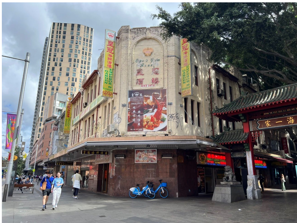
Figure 37 No. 100 Hay Street with its chamfered corner and arches and balustrades to the central and north bay to Dixon Street.
