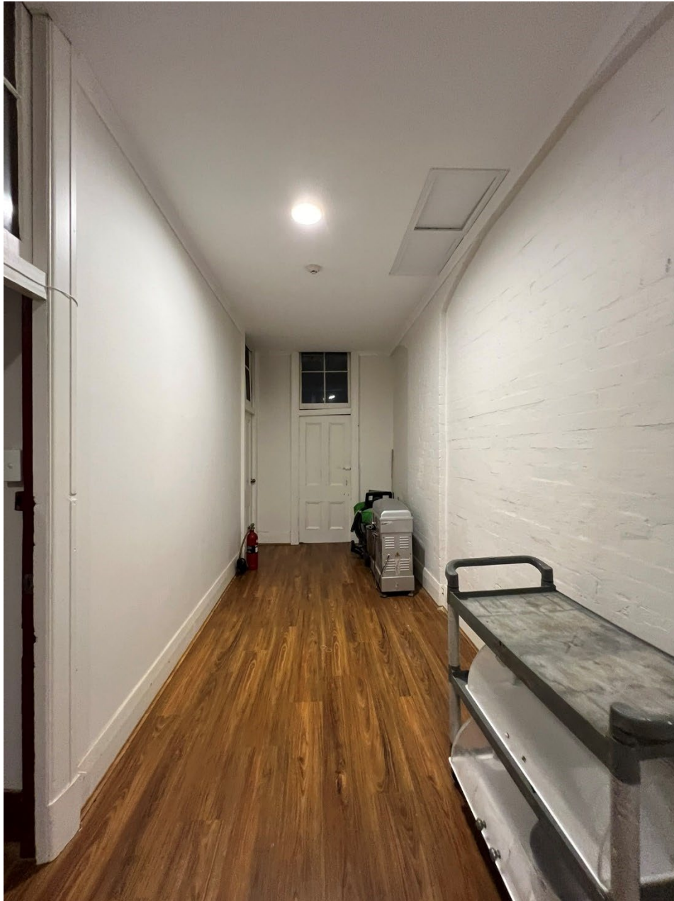
Figure 46 Second floor with 100 Hay Street with original joinery and recessed brick arches, false ceiling and modern floor boards.
